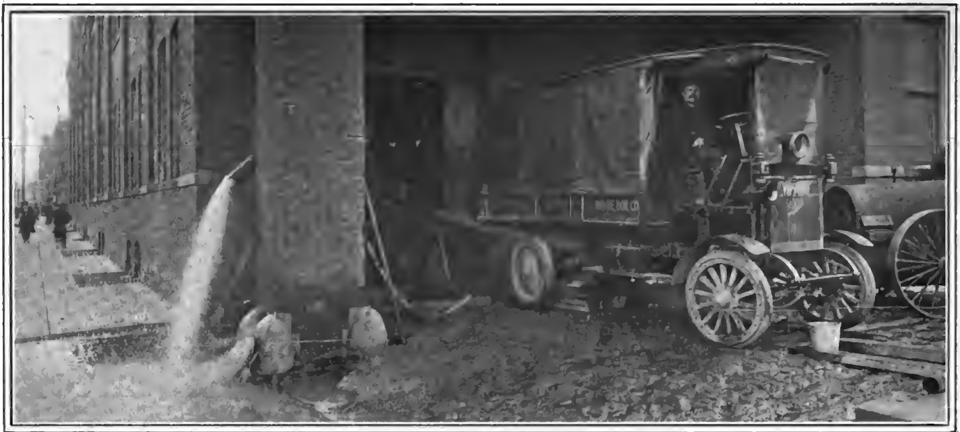
In Fort Wayne an Ideal motor truck was used to pump water out of a flooded building
